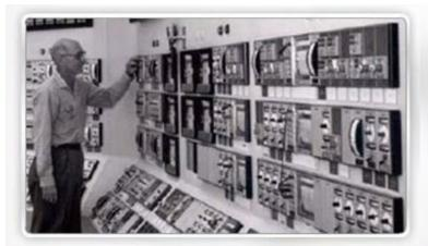
**Traditional control systems:** These control systems used banks of relays and contactors with no operator interface other than start or stop buttons to initiate actions and lamps to follow the progress of an operation and notify the operator upon completion.
